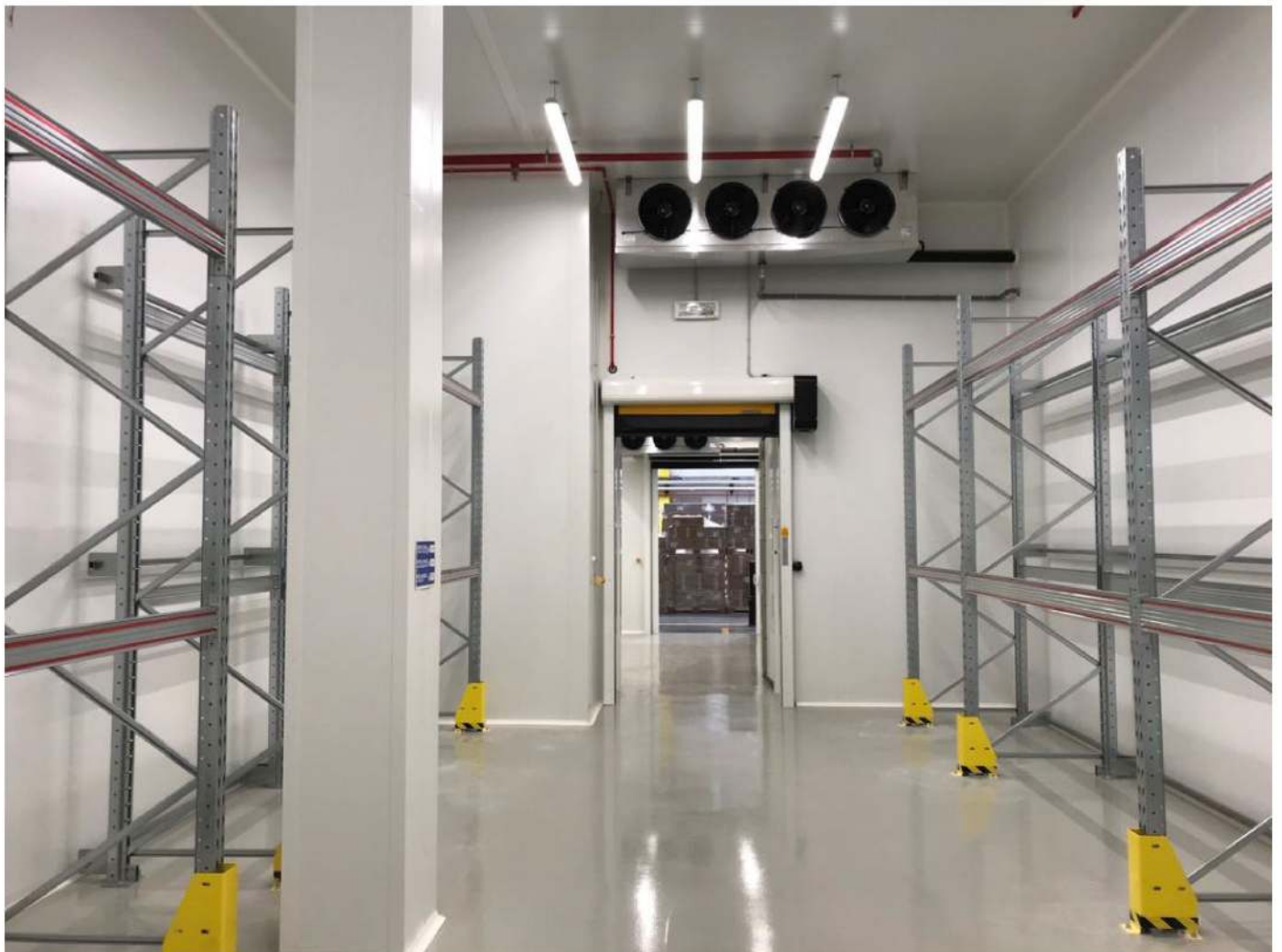
Example of Cold Room Interior:
