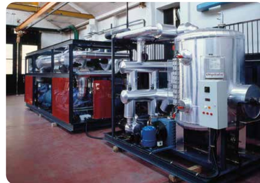
Brine package chilling units down to -75°C cascade system, equipped with pumps and liquid tank. Refrigeration system for the production of antibiotics.
